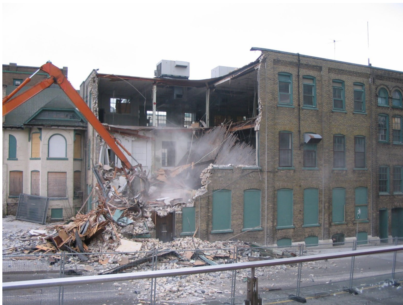
Demolition of the Forsyth Shirt Factory, Kitchener
