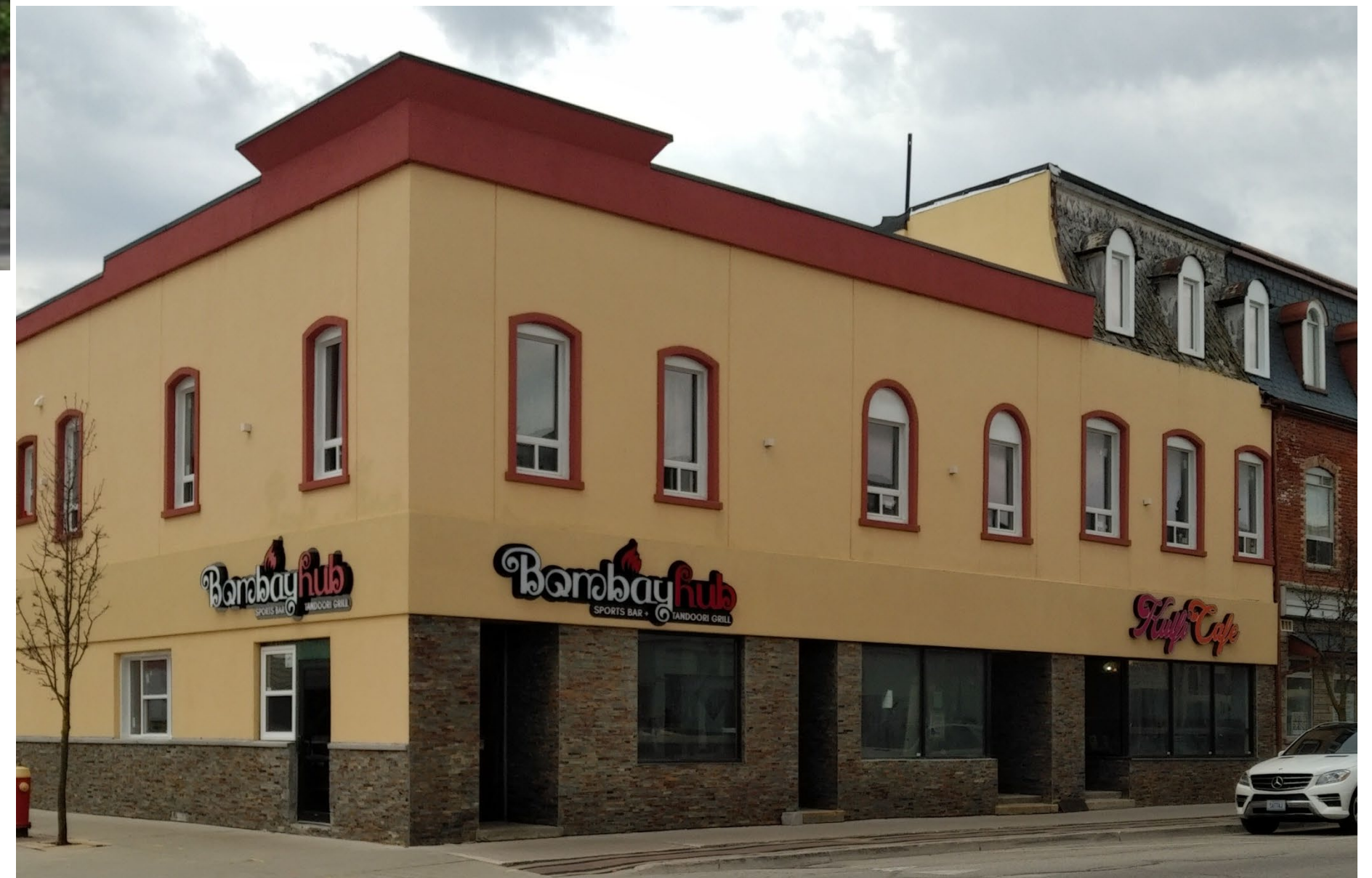
2023 Palmerston Main Street Refurbished and fully inhabited upper stories and stores = customers for uptown businesses.
